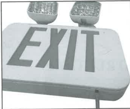
Remove the front cover
